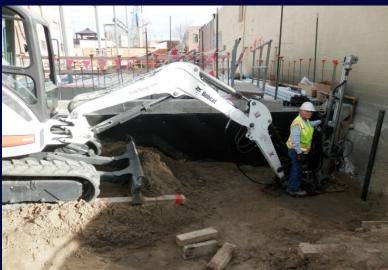
Park Range Construction was contracted to install over 119 Magnum 3" Reinforced Tubular Helical Piers for the new restaurant foundation. The site required the operation of drilling rigs which could operate in tight quarters between two existing buildings.
