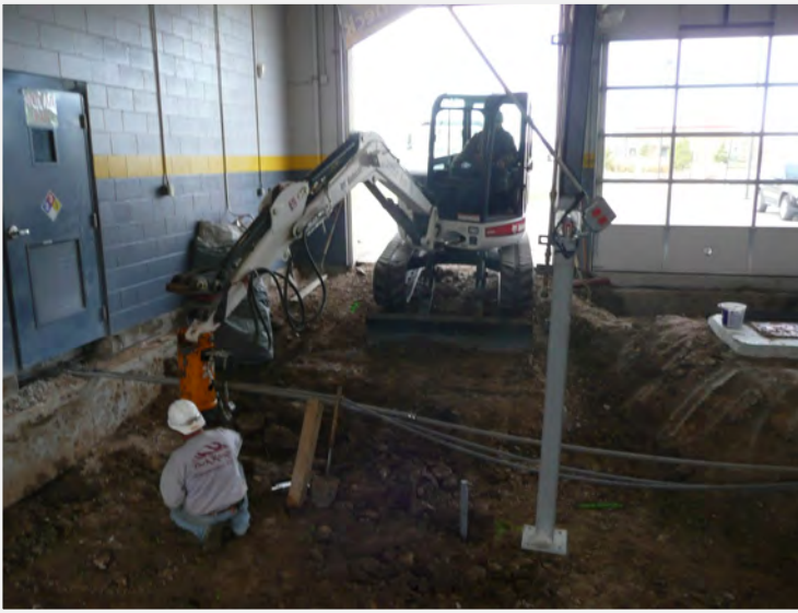
Photo: Installation of ECP 1-3/4" sq. galvanized helical piers to support vehicle alignment center and delicate lift column sensors.
