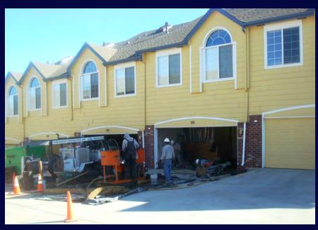
dation, revoiding of the foundation along the length of the porch walls as well as replacement of concrete porch slabs.
