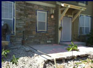
The HOA community had numerous issues with spalled and cracked concrete porches. The railings and columns originally designed did not allow for water to drain and the wooden columns were rotting. See Wood/Stone/Veneer Before photo at upper left. This community-wide project involved concrete demolition, pipe re-direction, railing and column re-design, rail to siding connections, rail abutment to stone walls, new wood columns with stone wrapping, flashing of
