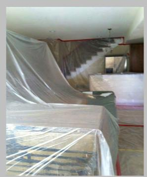
Park Range provided floor to ceiling containment to separate the finished basement from the upstairs living space during construction.
