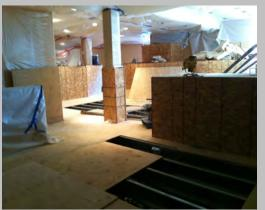
A Littleton home was experiencing buckling foundation walls and structural floors due to expansive soil pressures imposed on the structure. Park Range Construction was hired to build counterfort walls and to install micropiles, realign the foundation walls and
